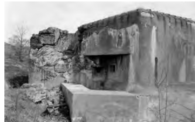
MO-S 19 Alej blockhouse at start of renovation process
