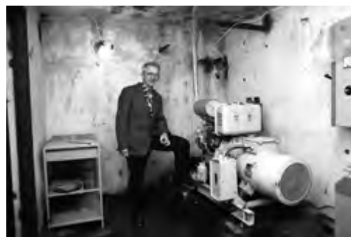
Jan Polášek next to generator in MO-S Alej, 1985
