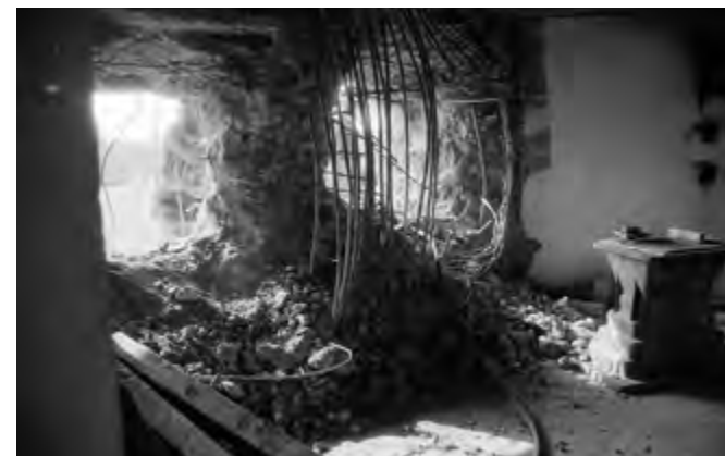
Right-hand shooting gallery before installation of embrasures
