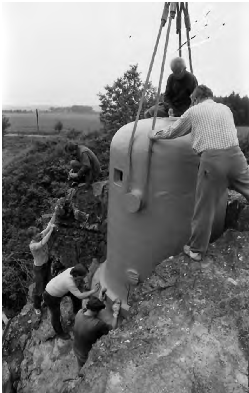
Installation of left-hand bell-chamber in MO-S 19 Alej (20 May 1986)
