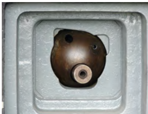
Detail of embrasure with sealing sphere
